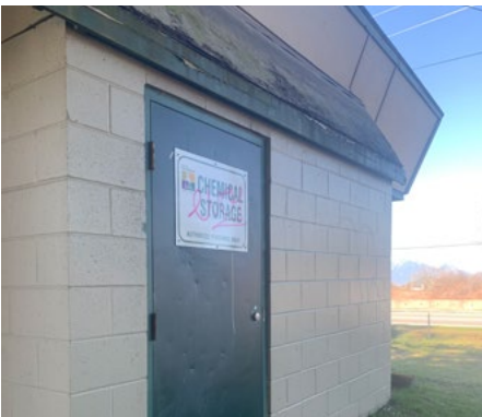
Chemical storage room
