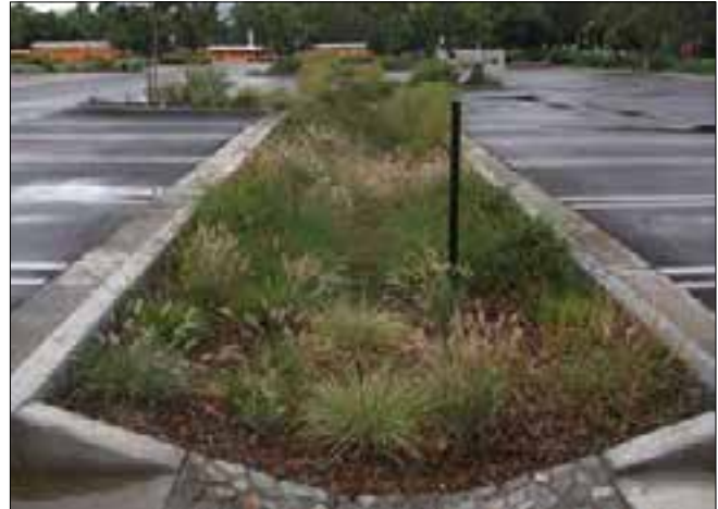
Planted island allowing surface water infiltration
